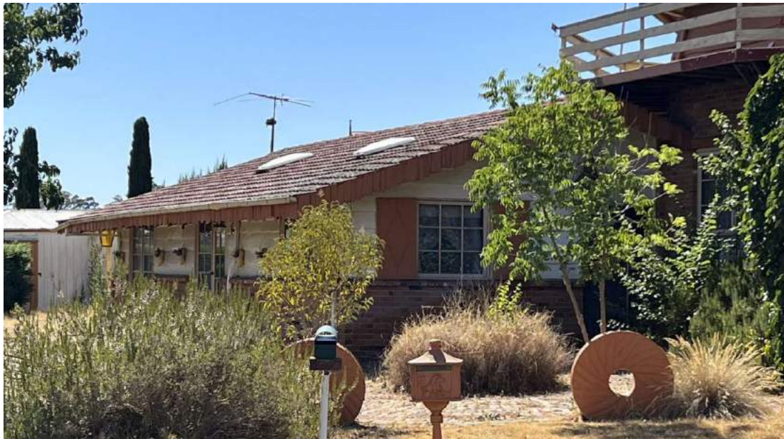
Figure 3: The single-storey wing to the north of the main windmill section. Note the brick to sill height and irregular shingle fascia.
