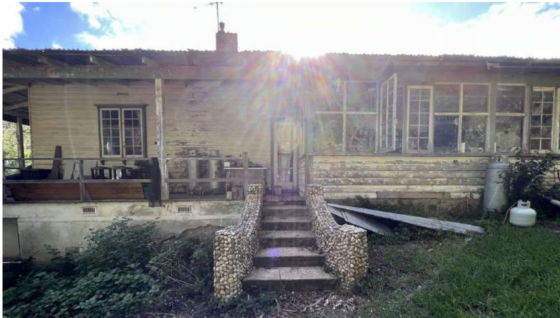
Figure 2: A view of the southwest of the house. The infilled veranda is visible to the right, and original or early pebble-detailed stairs central. Source: Trethowan 2022.
