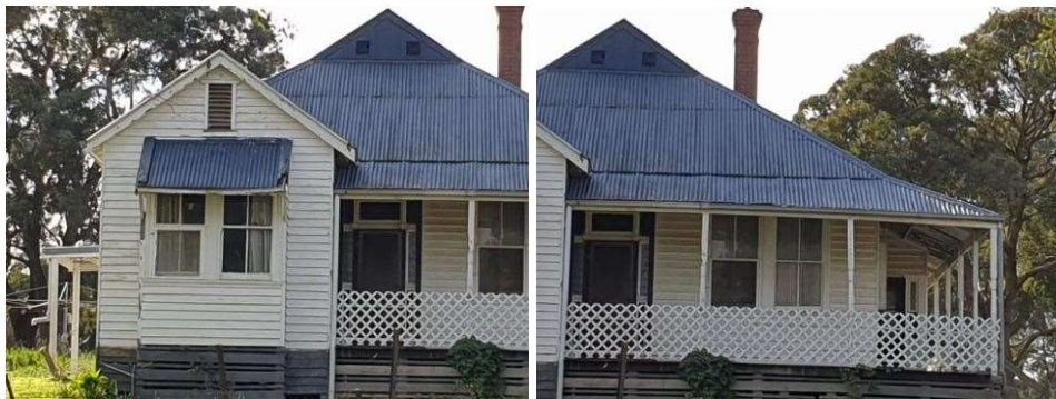
Figure 13: Façade of house at 14-26 Browns Lane, Plenty. Note the weatherboard construction. Source: Citation for 14-26 Browns Lane, plenty prepared by Context 2021.
