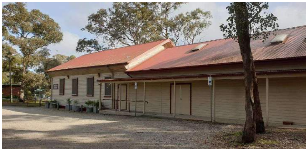
Figure 12. Eastern elevation of the Plenty Hall showing the taller original building built in 1930-31 and the lower extension added in 2010. (Source: Context June 2021).
