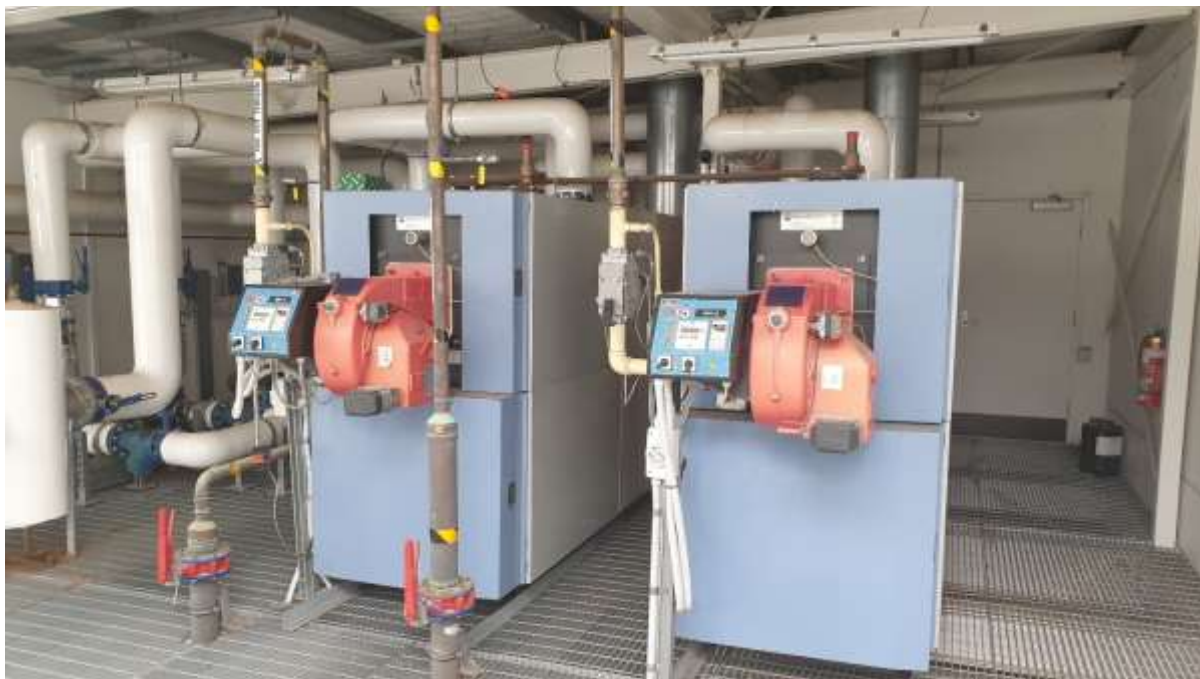
Figure 3: The two rooftop gas boilers at the Eltham Leisure Centre.
