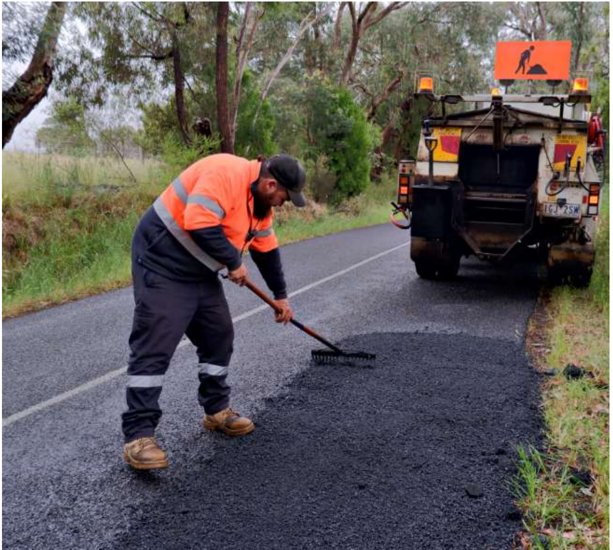
Image: Council's roads team repairing potholes in the Shire
