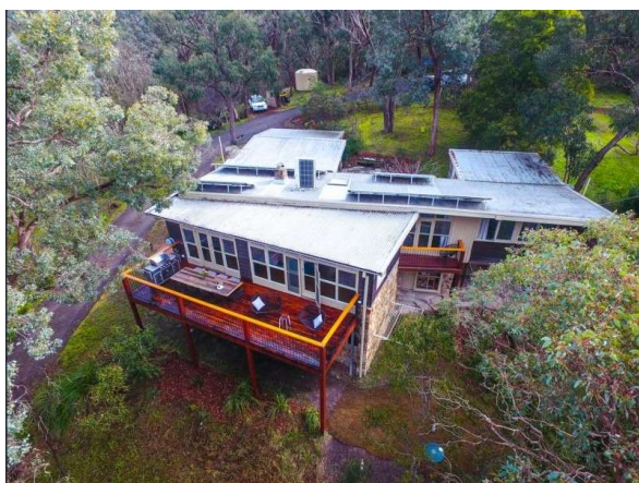
Figure 9: View of the south (front) elevation showing the later deck, the stone walls, and the roof form comprising butterfly and skillion components. Source: realestate.com.au, accessed March 2022.
