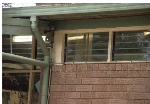
Figure 17. Detail of the glass louvred clerestory windows on the eastern side of the preschool (Source: Context 2020)
