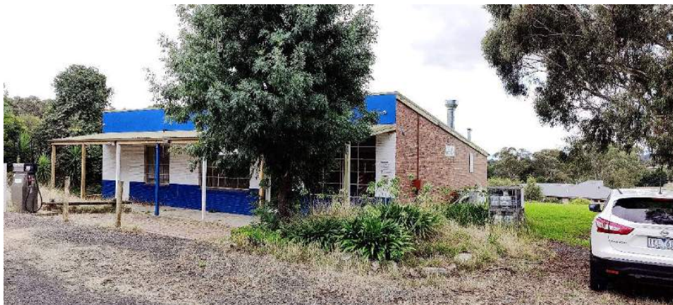
Figure 9: South (front) view of the shop. Note the skillion roof form and verandah. Source: Trethowan Architecture, 2022.
