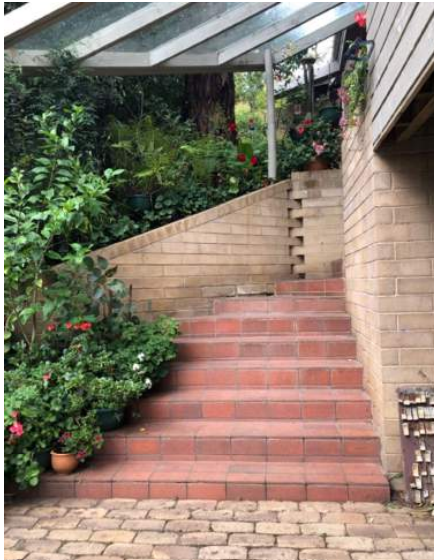
Steps from carport to secondary front entry, showing brickwork, tiled steps and brick paving. Source: Trethowan Architecture 2022
