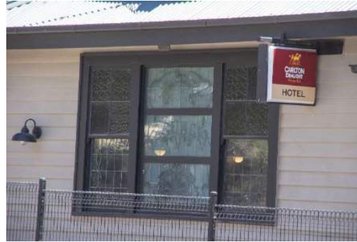
Figure 14. Tripartite bay window with leadlight and textured glass glazing. (Source: Context 2020)
