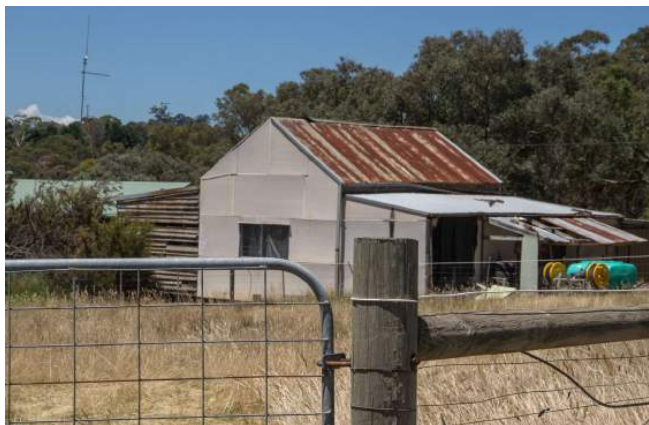
Figure 22. 191 Cherry Tree Road clad in painted sheets on the primary (south) and side (west) elevations. The window on the west elevation shown here and the verandah to the front of the house are later additions. (Source: Context 2020)
