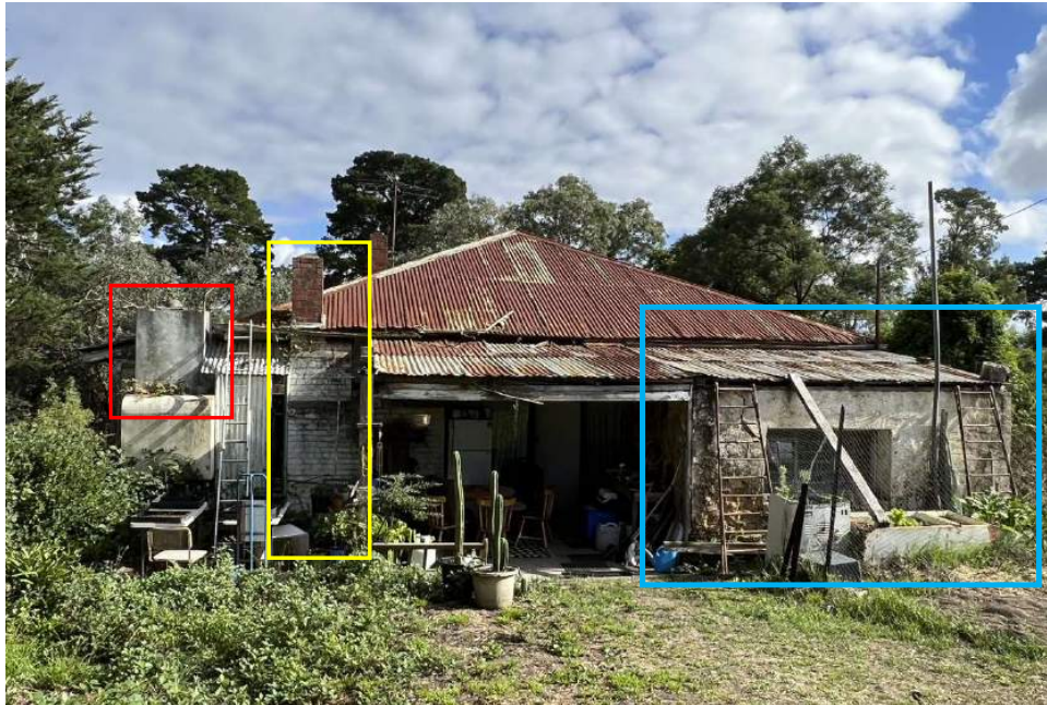
Figure 3: A view of the southeast of the house. The c1950s concrete chimney to the infill veranda room is highlighted in red; the original interwar kitchen chimney in yellow. The later stone rear addition is highlighted in blue. Source: Trethowan 2022.
