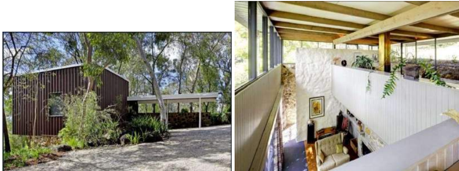
Figure: Views of the Wright House, note the use of exposed timber and stone internally, and the simple exterior form with skillion roofs. Source: realestate.com.au
