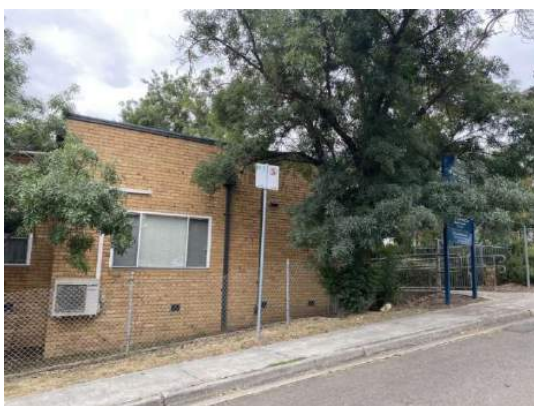
Figure 17. Southern elevation of former Eltham Infant Welfare Centre showing sheer unadorned wall surface of cream brick with low parapet concealing flat roof. (Source: Context, December 2020)
