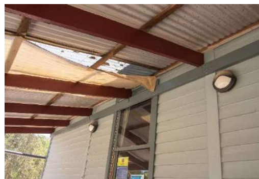
Figure 13. Window, corrugated iron and translucent polycarbonate clad verandah. (Source: Context 2020)
