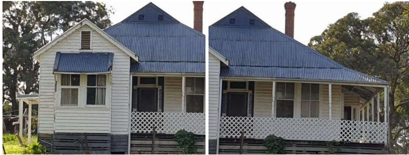
Figure 3: Façade of house at 14-26 Browns Lane, Plenty. Note the weatherboard construction. Source: Citation for 14-26 Browns Lane, plenty prepared by Context 2021.
