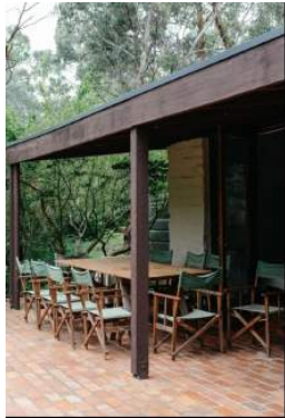
Figure 11: Photo shows the southern section of the rear (east) elevation of the 1972 section. Note the prominent timber columns and the wall of handmade bricks. Source: Airbnb.
