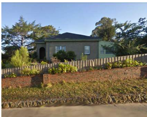
Figure 16. Secondary elevation facing Livingstone Road showing porch entrance arch, simple window detailing, and weatherboard rear extension. (Source: Google Streetview 2010)
