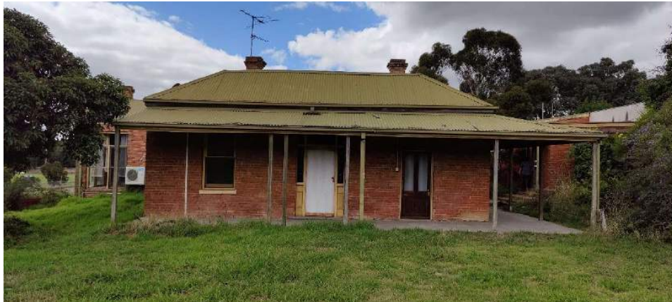
Figure 4: Front (west) elevation of the house. Note the original brick chimneys and the later door at the southern front room. Source: Trethowan Architecture, 2022.
