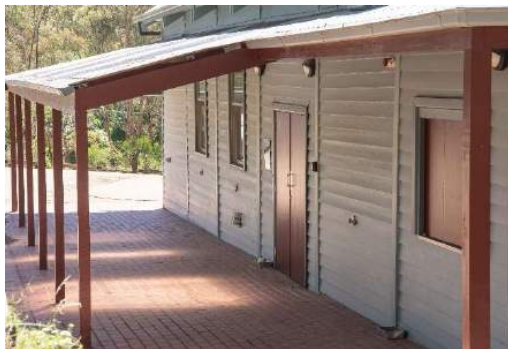
Figure 10. Corrugated iron verandah supported by timber posts over red brick paving. (Source: Context 2020)
