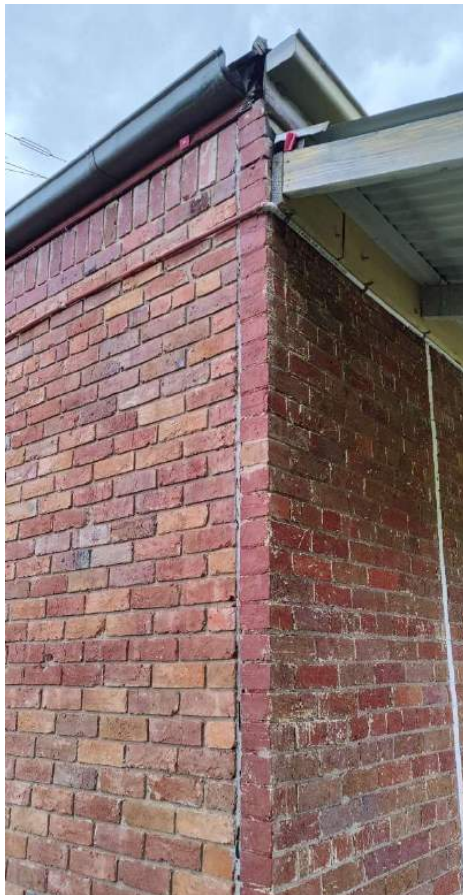
Figure 6: Joint between the new brick north wall (left) and earlier brick west wall. Source: Trethowan Architecture, 2022.
