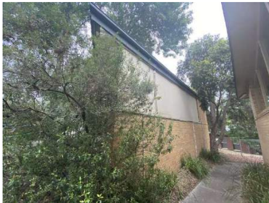
Figure 19. North elevation of the former Infant Welfare Centre showing dwarf closed wall above that was originally a louvred screen to pram porch. (Source: Context, December 2020)
