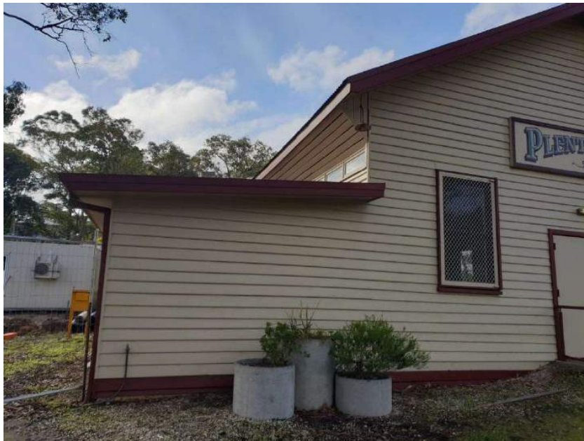
Figure 13. South west corner of the Plenty Hall showing the skillin roofed additions along the building westernside. Note the chamfered open slatted eave detail of the original Hall building. (Source: Context June 2021)
