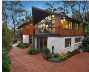
Figure 13 and Figure 14 show the dwelling. Note the mud brick walls, wide eaves and verandah and windows from floor to ceiling. Source: realestate.com.au, c2010s.
