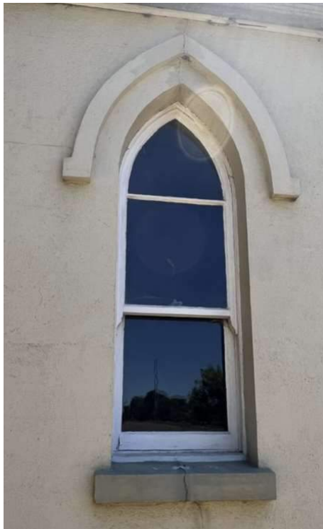
Figure 2: An example of an original side window with drip mould.
