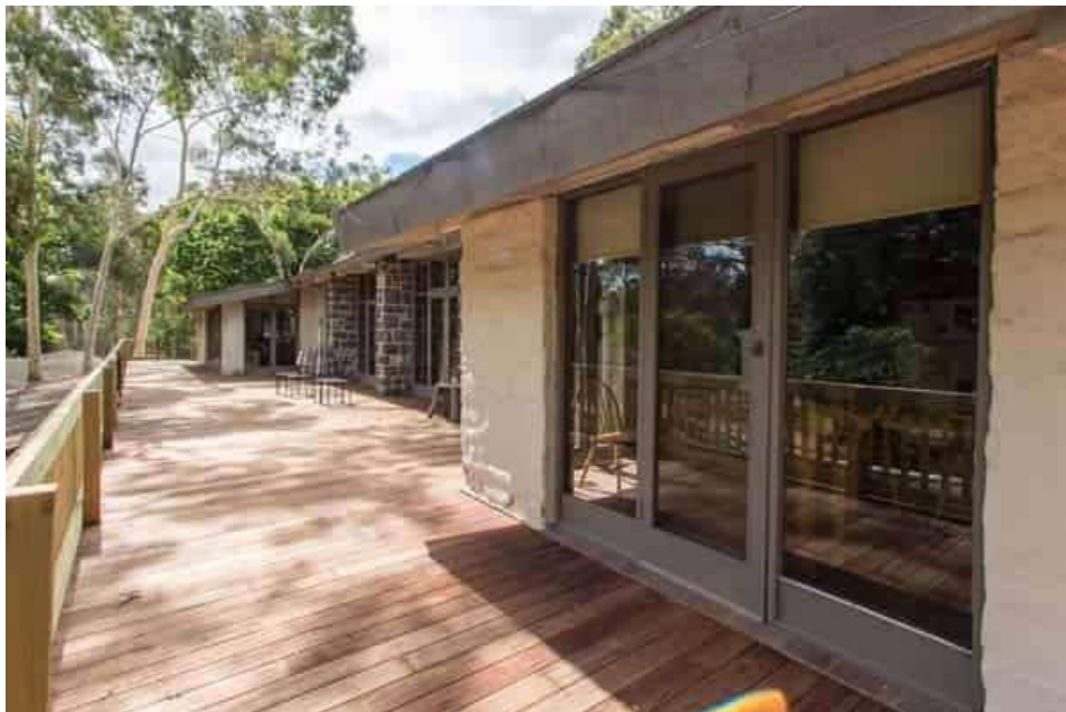
Figure 3: A view of the southern façade, showing the central recessed section with bluestone piers. Source: Tony Knox, Alistair Knox Foundation.
