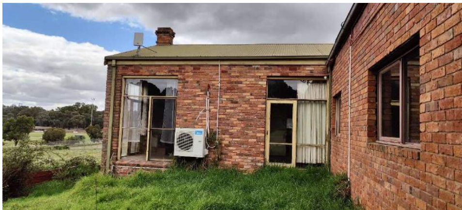
Figure 5: North elevation of the original house, looking east towards the rear extension. Note the matching brick wall cladding and roof sheet between the original and later parts of the house. Source: Trethowan Architecture, 2022.
