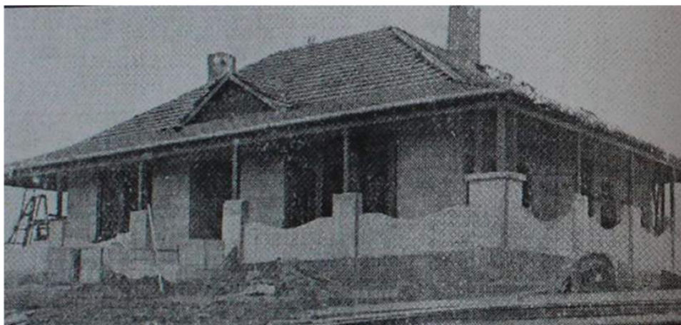
Figure 1: A view of the principal facade of the Perversi house under construction c1924, taken from the southwest. Note the chimneys, curved balustrade and small gable. Source: Bates 2006:36.
