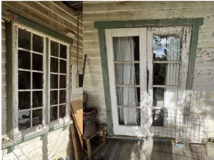
Figure 4: Examples of the casement windows (left) and French doors (right) with timber surrounds evident across the building. Source: Trethowan 2022.
