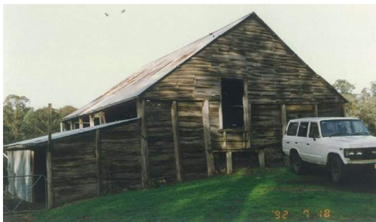
Figure 4: Drop-slab barn at Cleir Hills in 1992. Source: Bick, Shire of Eltham Heritage Study , 1992.
