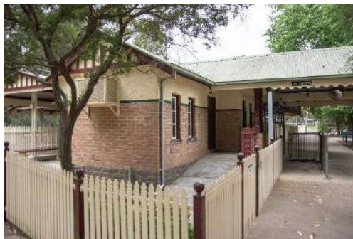
Figure 6. Station building with scalloped fascia. (Context 2020)
