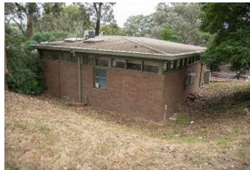
Figure 13. Rear of the infant welfare pavilion showing clerestory windows and a double hung window. (Source: Context 2020)
