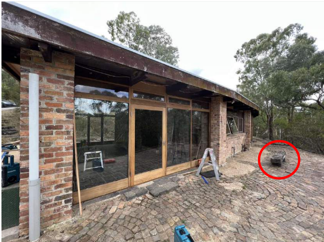
Figure 4: The south of the house, showing how the sets of doors and windows are set between brick columns. Note the stained fascia, shell pattern brick paving and bluestone bench (highlighted in red). Source: Trethowan Architecture 2022.
