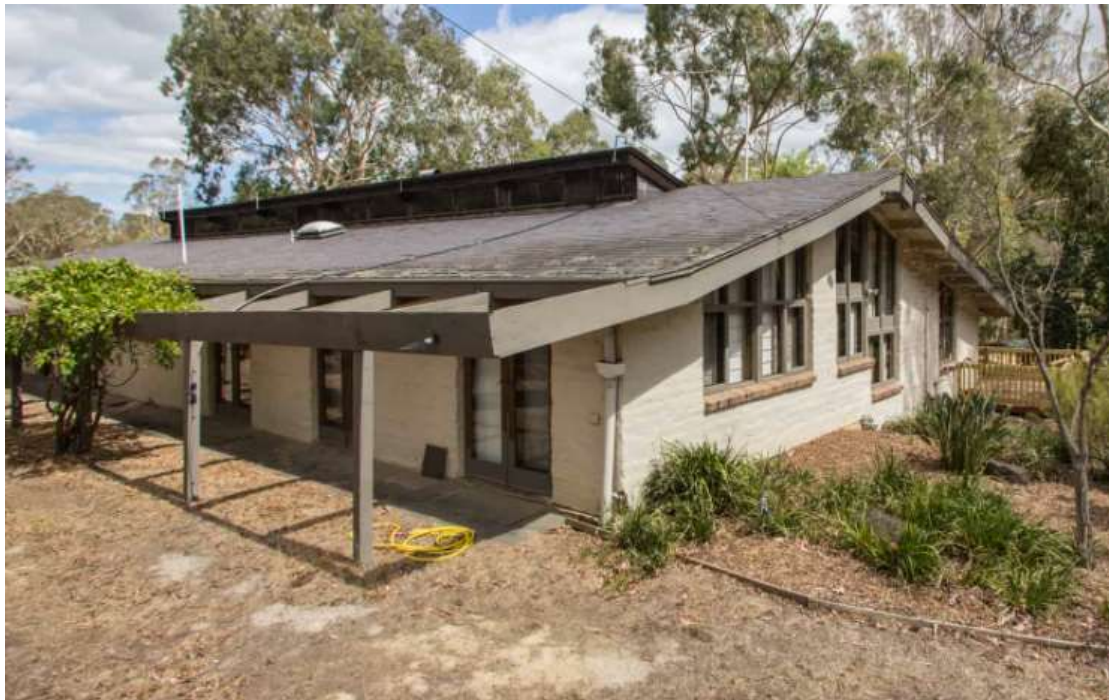
Figure 4: A view of the north east of the house. The original rafters extending to create the trellis on the north are still evident in this photo but have been removed. Note the clerestory windows. Source: Tony Knox, Alistair Knox Foundation.
