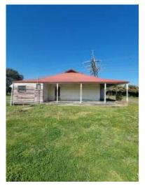
Figure 15. North elevation showing the return verandah with turned timber posts and Dutch gable end. (Source: Nillumbik Shire Council, photograph of owner)
