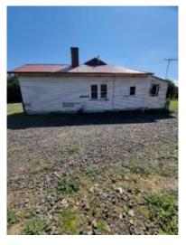
Figure 16. South elevation showing Dutch gable end, red brick chimney, pair of double-hung sash windows. (Source: Nillumbik Shire Council, photograph of owner)
