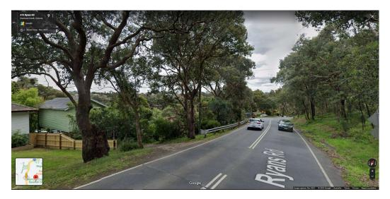
Figure 10: Example of existing roadside conditions at 417 Ryans Road Diamond Creek (Google Street View looking north, west on left hand side, east on right hand side), showing a constrained ability to provide a footpath on the western side of Ryans Road due to vegetation and topography
