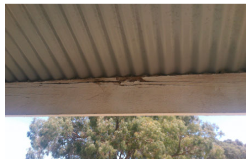
10. Water-damaged verandah beams
