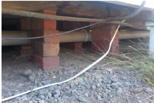
11. Floor bearers supported on bricks
