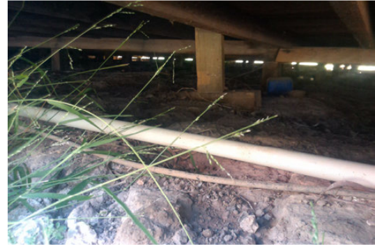
12. Floor bearers supported on props
