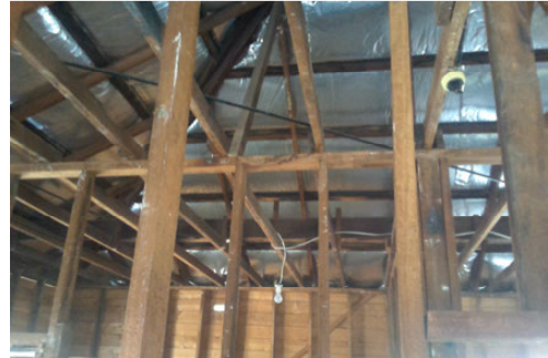
6. Roof strut not adequately supported
