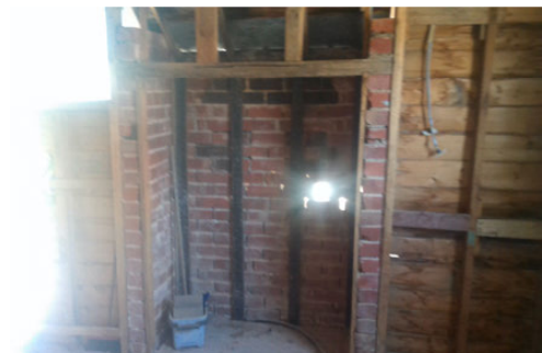
8. Single skin brick wall not braced
