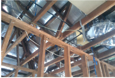
5. Roof strut not adequately supported
