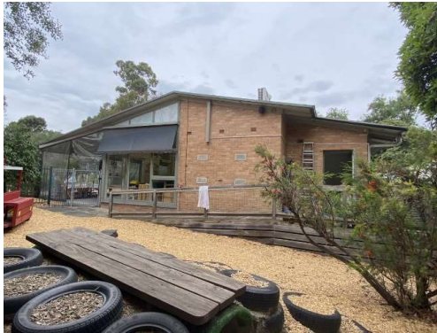
Figure 25. North elevation of the preschool building showing window wall, low-pitched gable roof and stepping in of building. (Source: Context, December 2020)
