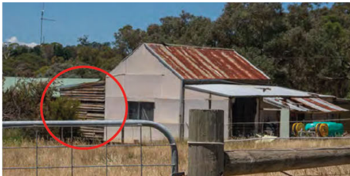
Figure 2. The original weatherboard cladding (circled) can be seen in terrible condition, missing pieces in various locations. The gabled roof is extremely rusted, with holes throughout.
