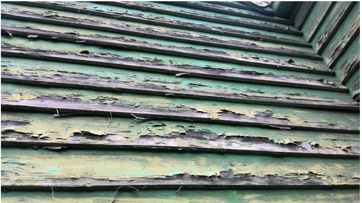
Typical Weatherboard Deterioration
