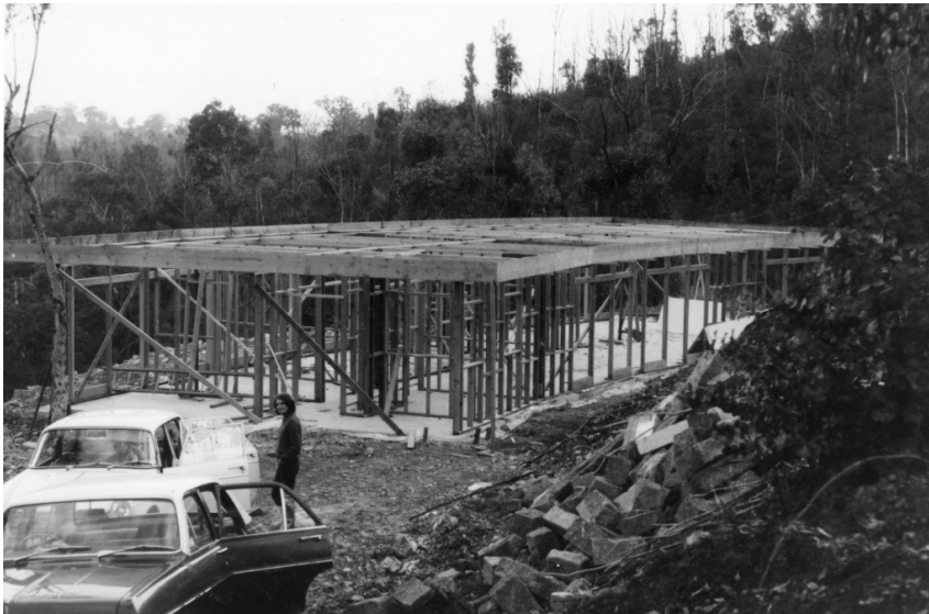
Figure 1: The house during construction c1968, showing its timber framing. Source: Cuming family, pers. Comm., January 2022.
