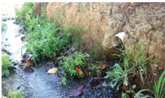
Figure 1: Greywater discharge to street culvert in Howell Road, Plenty
