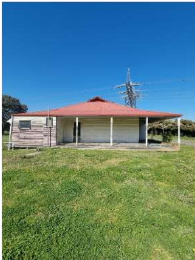
Figure 15. North elevation showing the return verandah with turned timber posts and Dutch gable end. (Source: Nillumbik Shire Council, photograph of owner)
