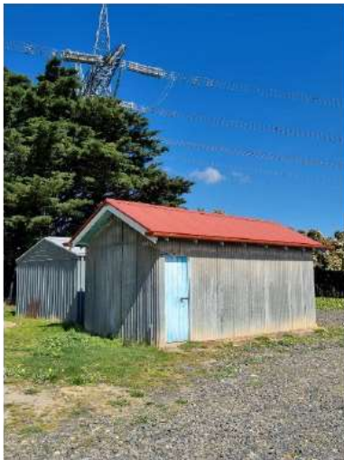
Figure 19. Timber garage with pitched roof and corrugated iron walls. (Source: Nillumbik Shire Council, photograph of owner)
