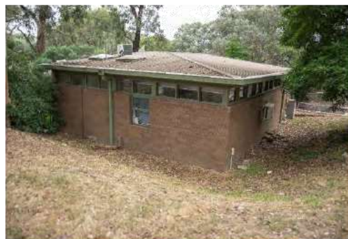
Figure 13. Rear of the infant welfare pavilion showing clerestory windows and a double hung window. (Source: Context 2020)
