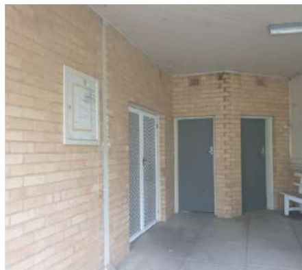
Figure 20. Pram porch at the former Eltham Infant welfare Centre. The two doors set on the angle provide access to bathrooms whilst the pair of doors to the left are the main entry to the building. (Source: Context, December 2020)
