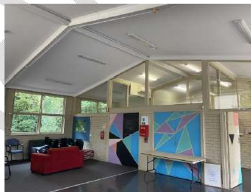
Figure 33. Interior of War Memorial Hall showing extant glazed partitioning system and expressed structural steel portal frame. (Source: Context, December 2020)
