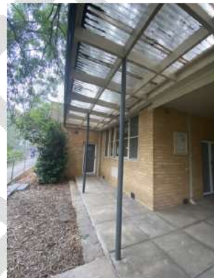
Figure 18. Pergola across principal elevation of the former Eltham Infant Welfare Centre showing slender metal posts. (Source: Context, December 2020)
