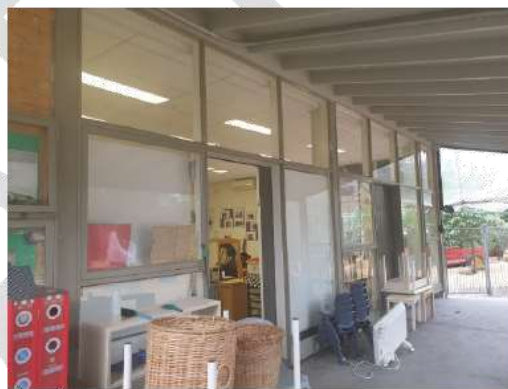
Figure 28. Window wall under verandah. Note the original eave overhand has been extended to create a deep undercover play area. (Source: Context, December 2020).
