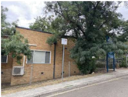
Figure 17. Southern elevation of former Eltham Infant Welfare Centre showing sheer unadorned wall surface of cream brick with low parapet concealing flat roof. (Source: Context, December 2020)
