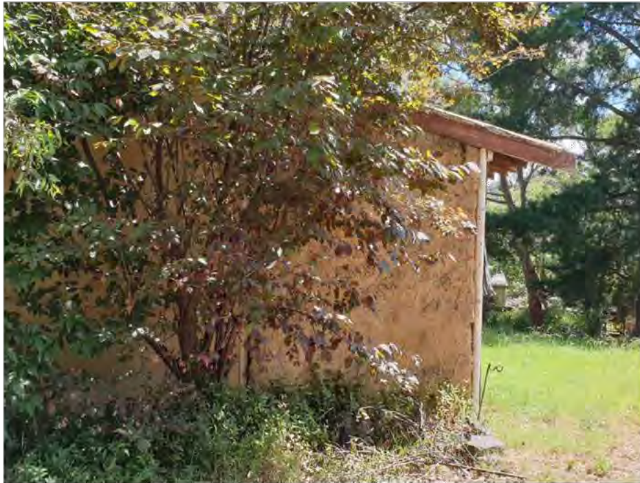
Figure 14. Southern wall of the bungalow that is constructed out of mudbrick for its eastern half and stud framed for the remainder. This elevation is visible from Park West Road. (source: Context 2020)
