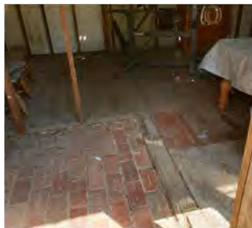
Figure 16. Detail showing the brick floor and evidence of an earlier stud wall forming an entrance porch. (Source: Context 2020)
