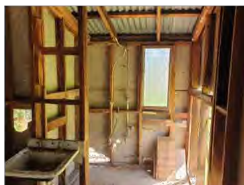
Figure 18. North east corner of the bungalow which housed the original bathroom evidenced by remnant plumbing fittings and fixtures. (Source: Context 2020)
