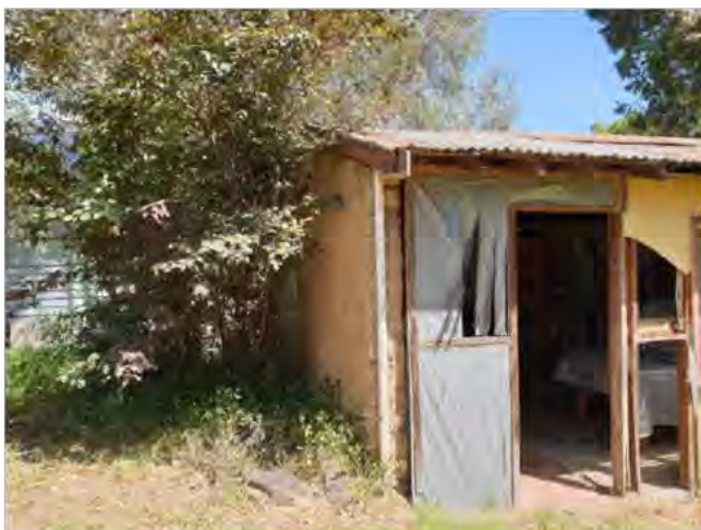
Figure 12. Section of eastern wall clad in grey that appears to have been added enclosing a small, recessed porch. The brick paved floor of the porch remains and there is evidence of the stud wall internally that housed the original front door as shown in Figure 8. (Source: Context 2020).
